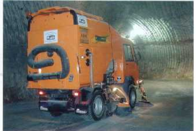
Sweeping machines in operation below ground
